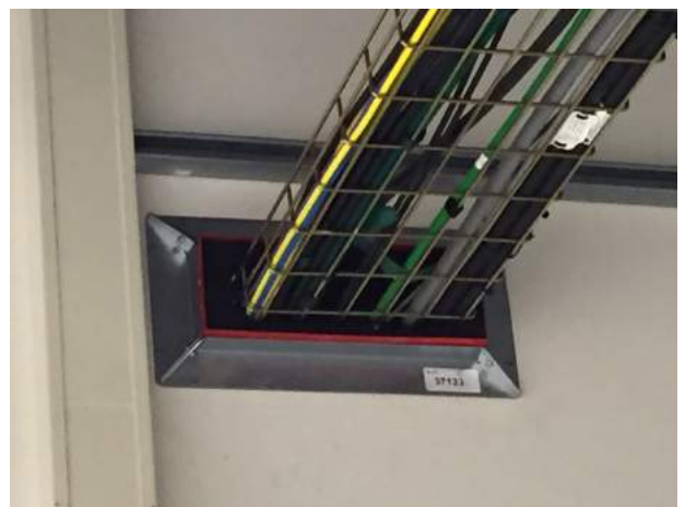
BB350 Box installed with flence
